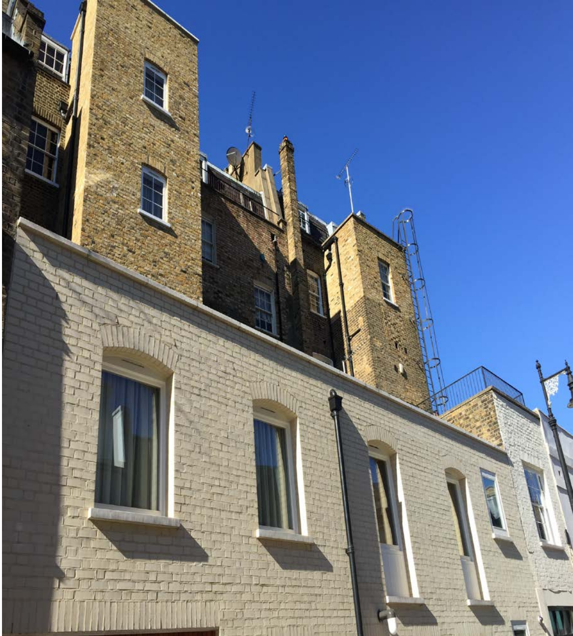
Front elevation of Nos. 44-45 Ebury Mews. The terrace is to be located on part of the roof of this property.
